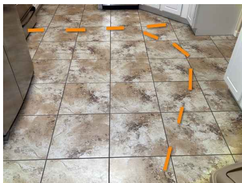
Kitchen overview of cracks
