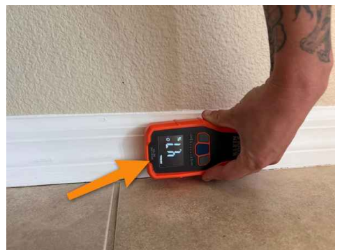
No elevated levels of moisture present
