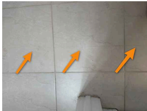
1st Hall Bathroom Hall
