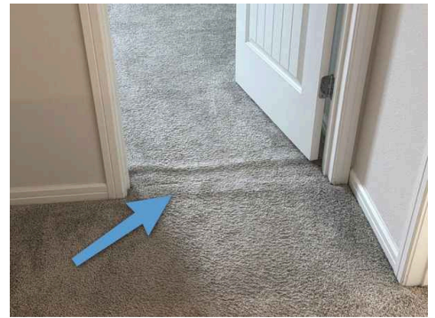
2nd Floor Hall
