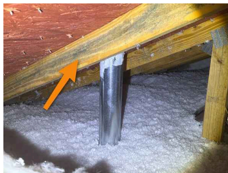
2nd Floor Attic
