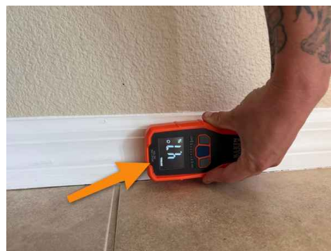
No elevated levels of moisture present
