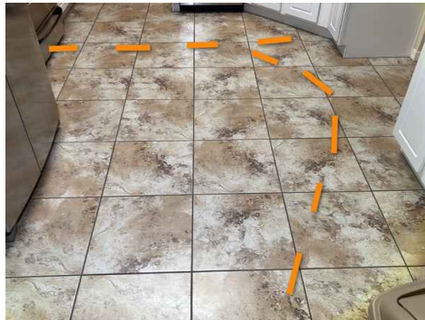
Kitchen overview of cracks
