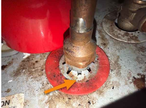
Entry Hall Closet
