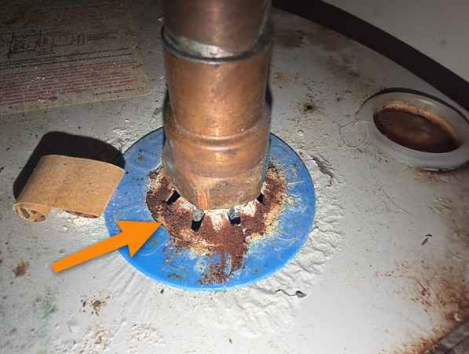
Entry Hall Closet
