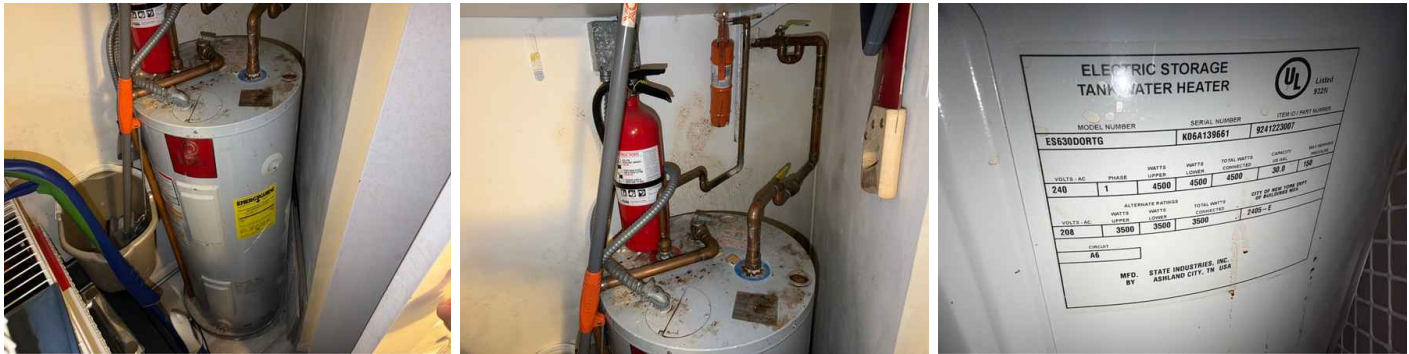
Entry Hall Closet
