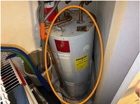
Entry Hall Closet
