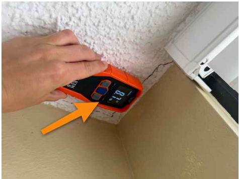
Dining- no elevated levels of moisture
