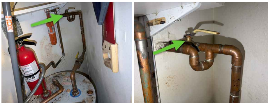
Entry Hall Closet
